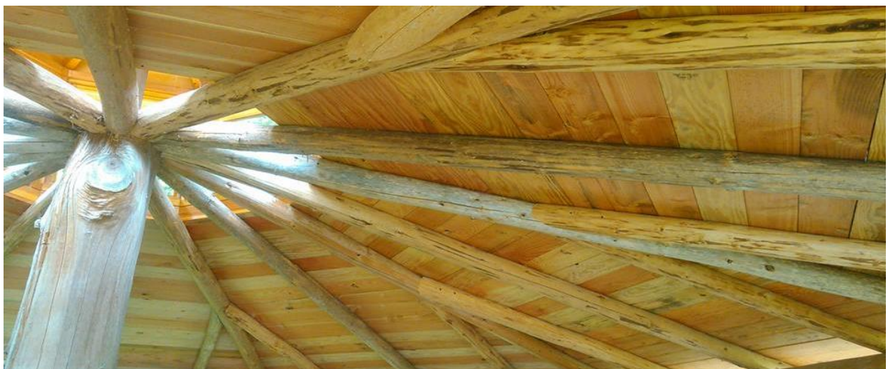
A gazebo constructed from small poles thinned from San Juan County forests. Photo: NNRG
