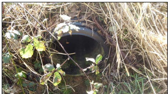
16" corrugated plastic culvert beneath northern access road.
