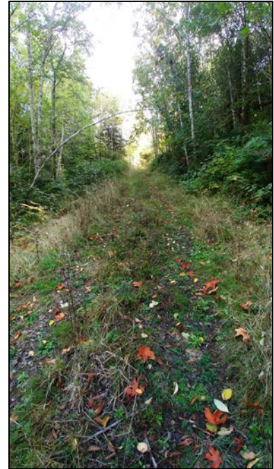
Forest access road up northern slope with light gravel surfacing, erosion and grasses on surface.
