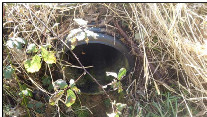
16" corrugated plastic culvert beneath northern access road.
