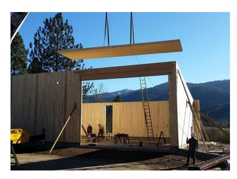
CLT wall and roof panel being hoisted into place at California's first all CLT building in Quincy, CA
